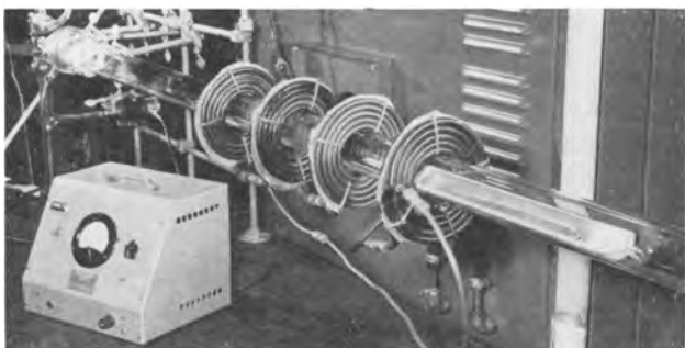
Fig. 2. Multiple-coil arrangement for zone melting
